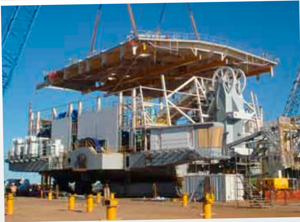
Successfully lifting the dragline's roof into place at Capcoal.
