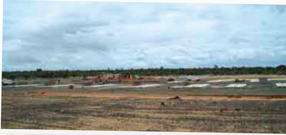
Construction of the Moranbah North Power Station has commenced.
